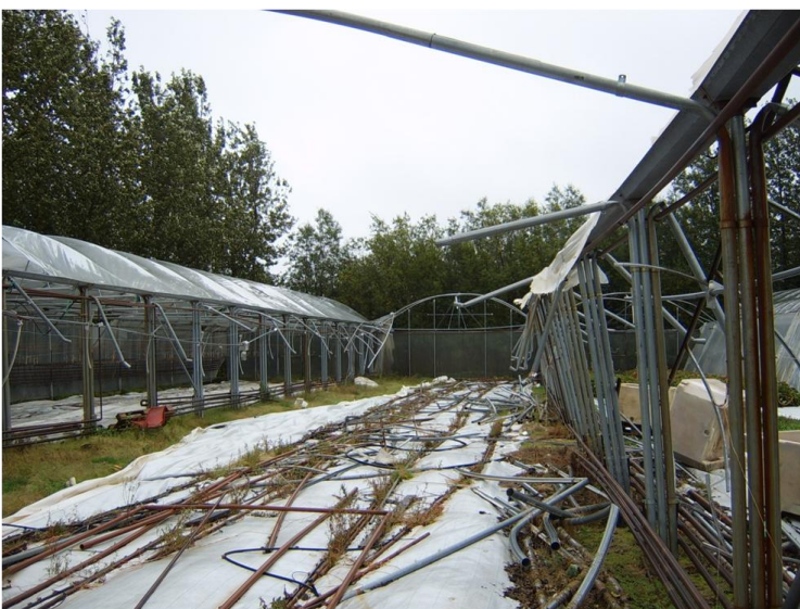
Figure 19. Damage to plastic house in Iceland due to snow pressure. Photo: Magnús Ágústsson
