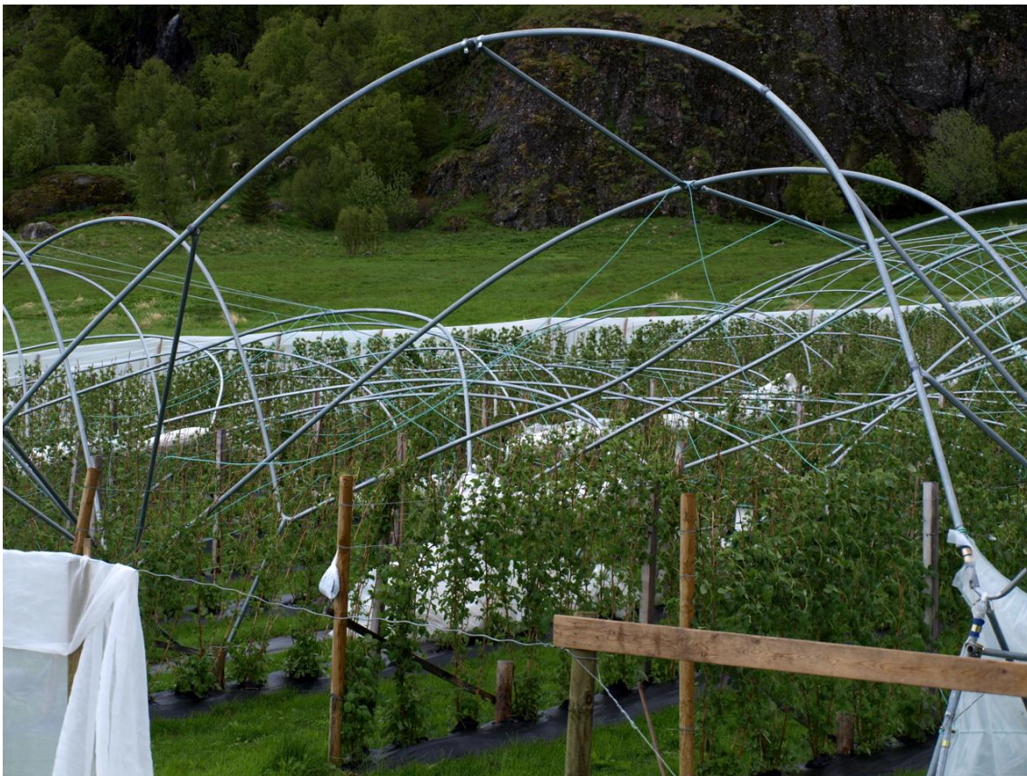
Figure 10. Wind damage to plastic tunnels by a storm 28 May 2009 at Grytøya, Norway. The tunnels are now replaced by a reinforced version of the Arctic tunnel. Photo: Pål Alvereng
